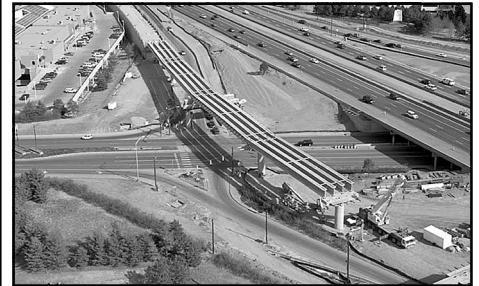
The new RTD Light Rail bridge under construction over Orchard Road. – Photo © Gregg Gargan, CDOT.
